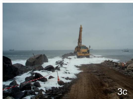
Figure 3: Setup 3D model (3a); The transition after 3D model testing (3b) and overtopping at the transition during construction (3c).
